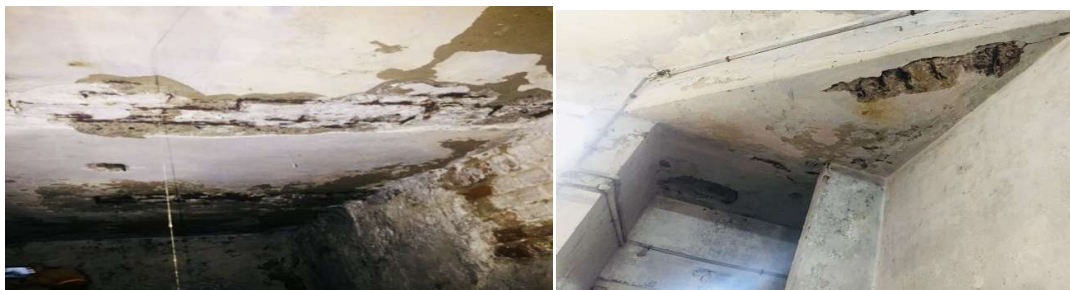
Fig.4 Spalling & Corrosion of reinforcement in structural element
